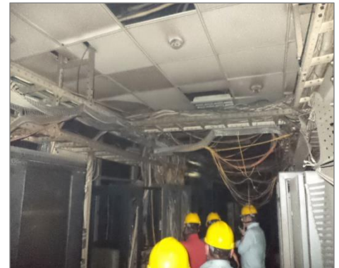
(f) Fire Safety Evaluation of PTCL Building
