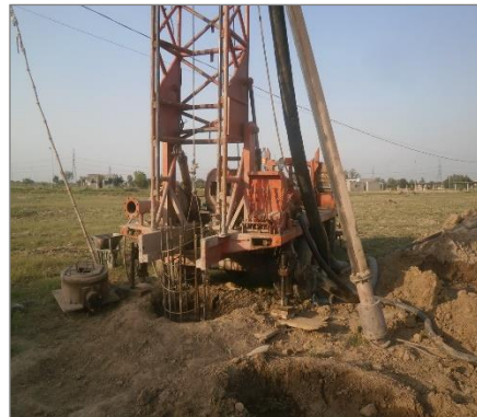
(e) Boring in ground for Soil investigation
