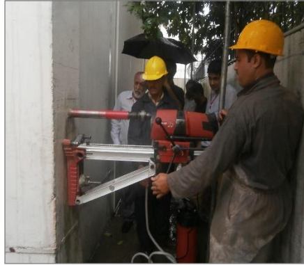
(b) Concrete Coring
