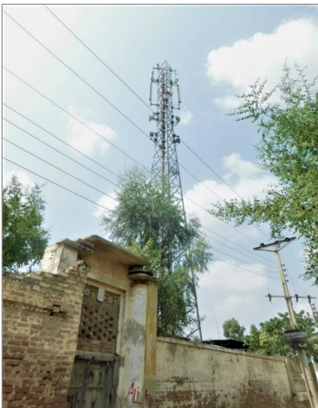
(a) Telecom Site Tower
